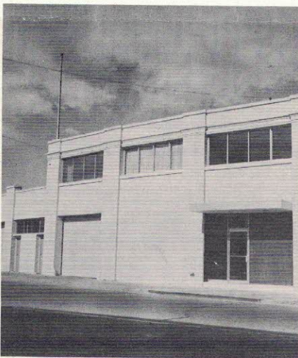
Renovated offices increase efficiency.
